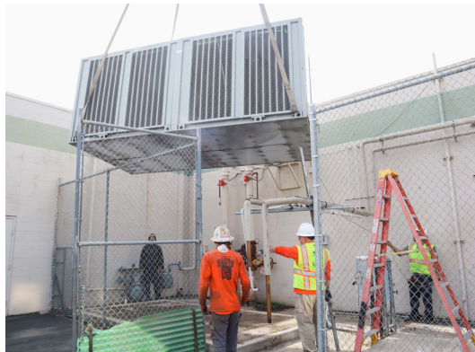
Replacing the condensing unit
