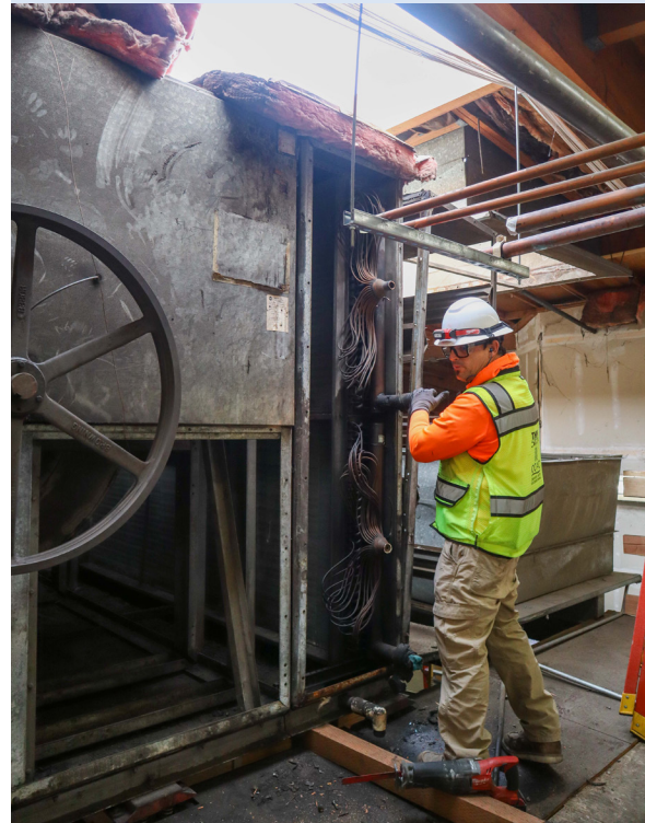
Bringing in the evaporator section through the temporary roof opening.
